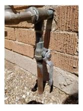
If the house does not have one there is a water meter box that also contains a main shut off valve. The meter box will be outside near the street or in the alleyway in the back.
