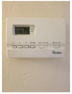
Set the "Heat-Cool" switch to COOL. Set the fan switch to AUTO. Then select the desired temperature. The AC requires a clean filter to operate efficiently. The filter is located under the furnace or air handler
