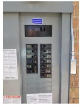
The main breaker will be 100A or 200A. This will shut down all electricity to the house. This is where you can turn off any circuit or full house in case of an emergency.
